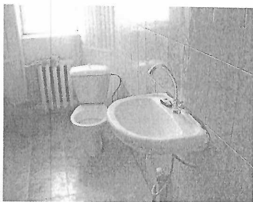
sanitary room after rehabilitation
