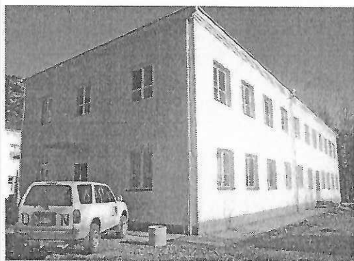
hospital building after rehabilitation
