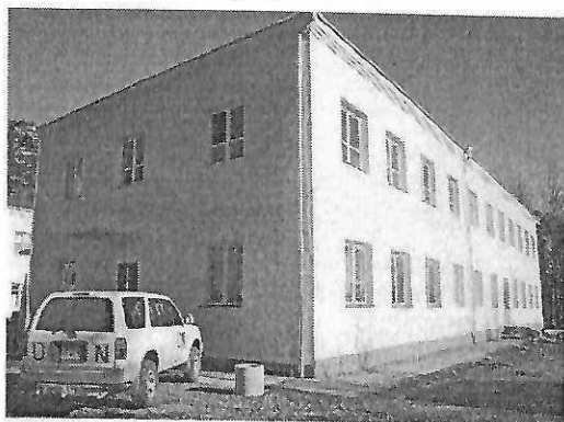
hospital building after rehabilitation
